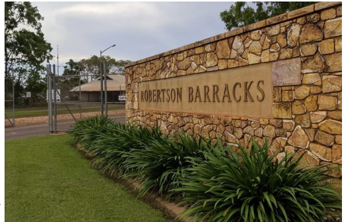
Robertson Barracks. From https://www.gjwalker.com.au/robertson-barracks .
